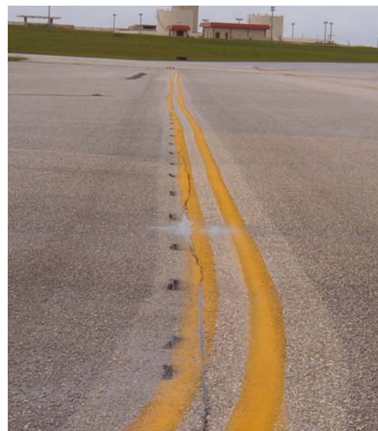
FIGURE 2-4. MARKING IS OUT OF ALIGNMENT
