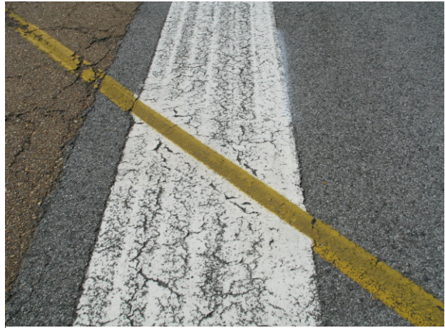
FIGURE 5-3. CRACKED AND PEELING MARKINGS – REMOVE 85 PERCENT.
