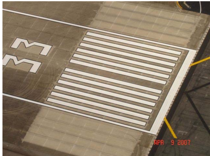
FIGURE 5-33. THE VISIBLE SCAR IS CLEANED PAVEMENT.
