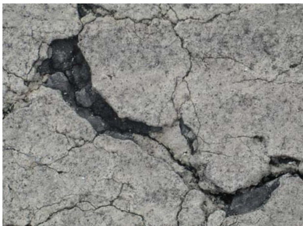
FIGURE 5-29. CRACKED PAINT INDICATES PRE-EXISTING PAVEMENT DETERIORATION.
