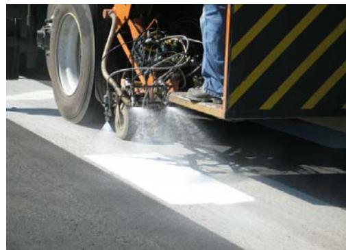
FIGURE 6-47. GLASS BEAD DISPENSERS ADJUSTED TOO HIGH.
