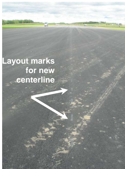
FIGURE 6-2. CONSTRUCTION DIRT MUST BE CLEANED.
