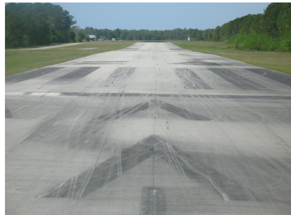
FIGURE 4-13. MARKINGS ARE OBSCURED BY ALGAE.
