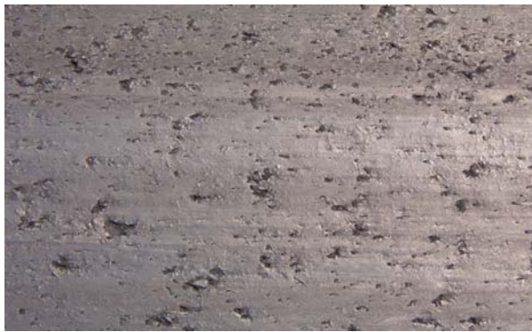
FIGURE 4-9. BEFORE RUBBER REMOVAL.
