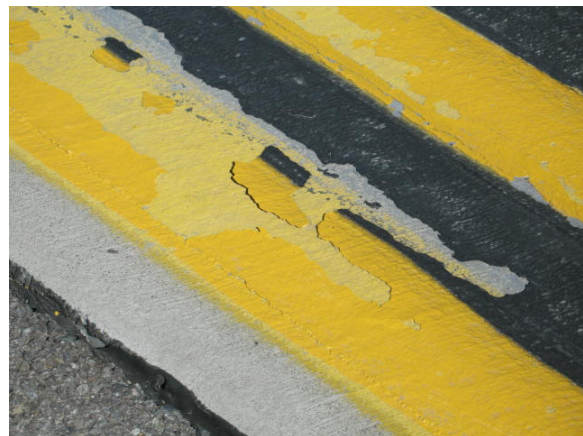
FIGURE 2-1. PEELING PAINT LAYERS
