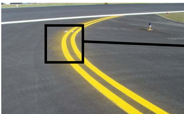
FIGURE 6-44. OVER SPRAY CAUSED BY WIND OR THINNED PAINT, OR BOTH.
