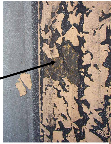
FIGURE 6-11. ENLARGED PORTION OF CRACKED ASPHALT.
