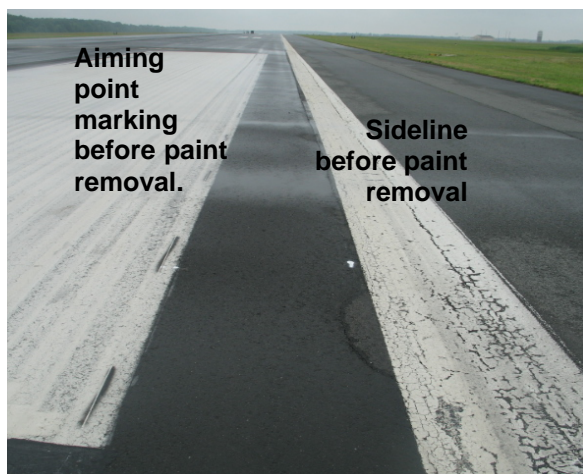
FIGURE 5-27. BEFORE PAINT REMOVAL. FIGURE 5-28. AFTER PAINT REMOVAL.
