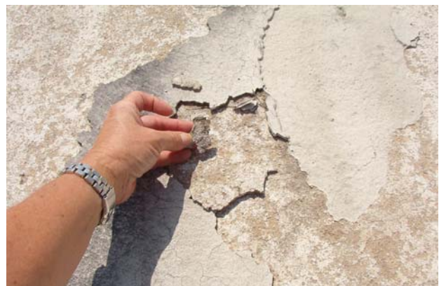
FIGURE 5-6. HEAVY PAINT BUILD UP ON CONCRETE.
