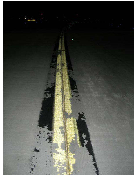
FIGURE 4-8. EXAMPLE OF POOR REMOVAL OF CURING COMPOUND.
