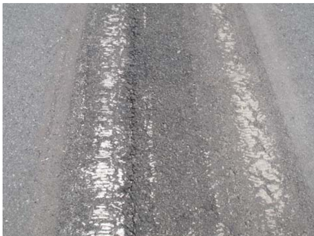
FIGURE 5-30. REMOVAL OF MULTIPLE LAYERS ON DETERIORATED ASPHALT.
