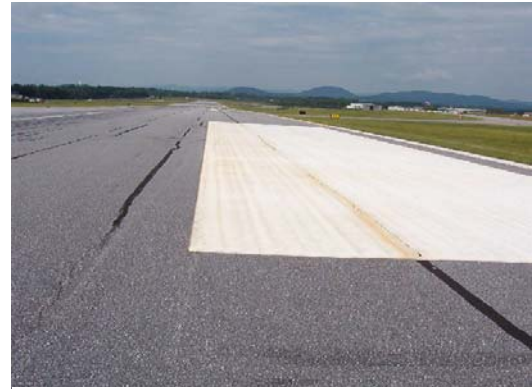
FIGURE 6-13. JOINT MATERIAL DISCOLORS THE WHITE PAINT.
