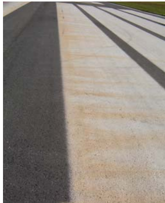
FIGURE 4-23. STAINED LEADING EDGE OF MARKING FROM IRON CONTAMINANTS.
