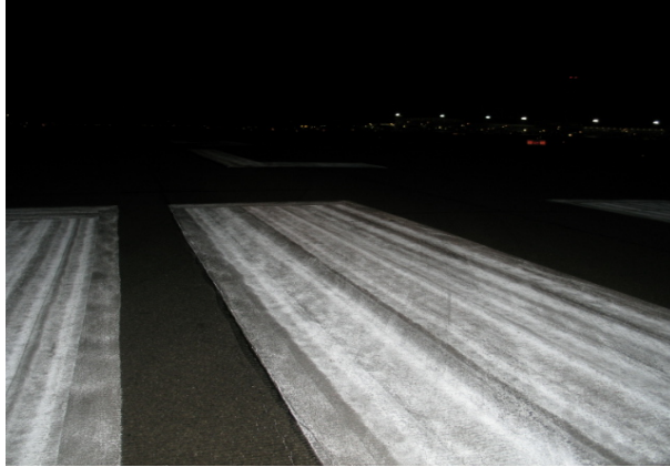
FIGURE 6-37. BORDER WAS APPLIED WITH HAND-MACHINE AND BEADS WERE HAND-THROWN.
