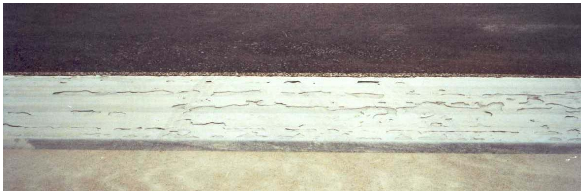
FIGURE 4-3. REPEATED PAINTING ON CONCRETE LEADS TO FOD.
