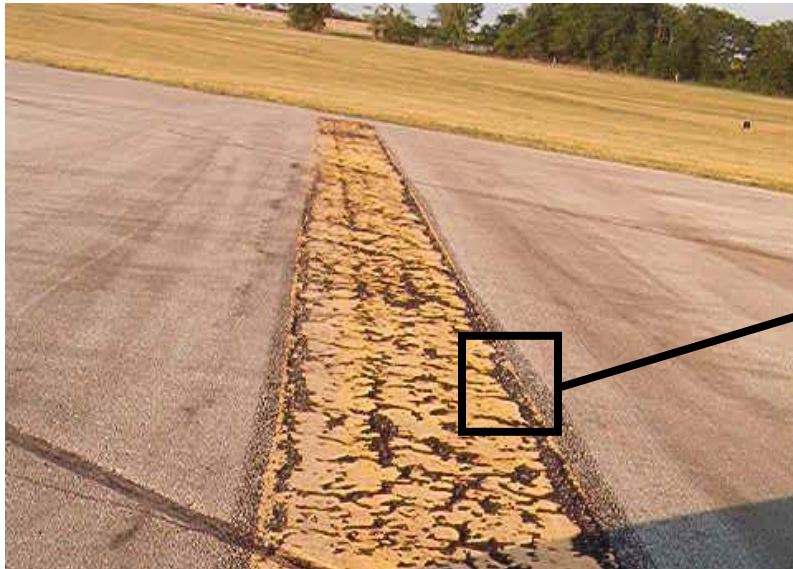
FIGURE 6-10. OLD SOLVENT PAINT CURLED, CRACKING THE ASPHALT TO WHICH IT WAS BONDED.
