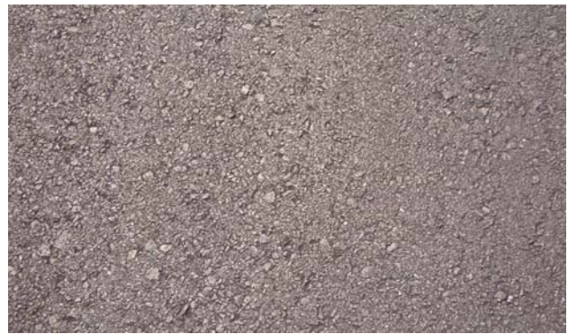
FIGURE 4-10. AFTER RUBBER REMOVAL.
