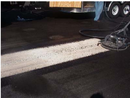
FIGURE 4-34. THE PROCESS USED TO REMOVE OIL STAIN.
