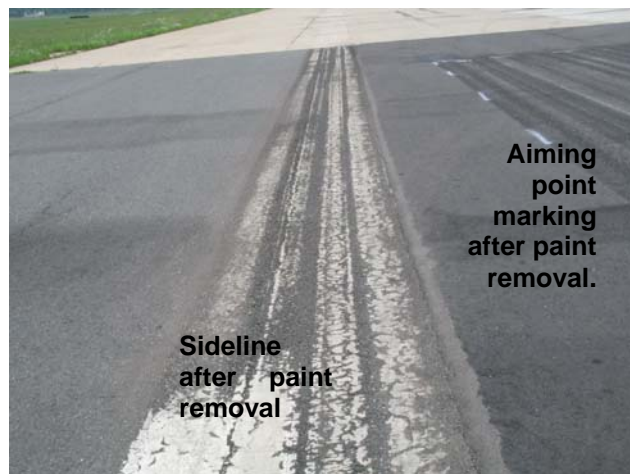
FIGURE 5-27. BEFORE PAINT REMOVAL. FIGURE 5-28. AFTER PAINT REMOVAL.
