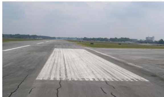
FIGURE 4-17. AFTER WATERBLASTING, BUT BEFORE PAINTING.
