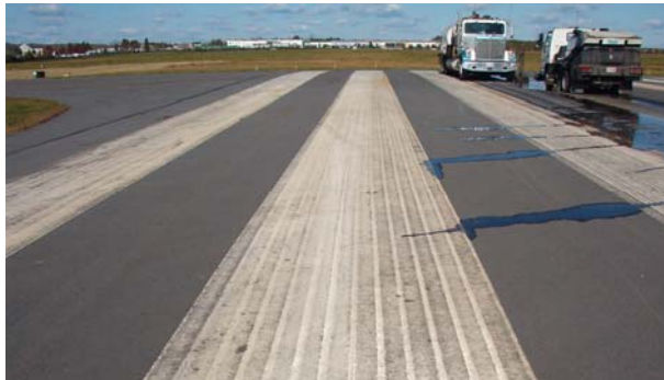
FIGURE 4-1. BEFORE CLEANING LOOSE AND POORLY BONDED PAINT.
