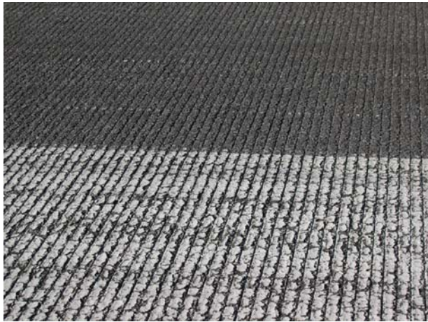
FIGURE 5-22. MARKING BEFORE (BOTTOM) AND AFTER (TOP) REMOVAL.
