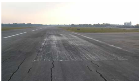
FIGURE 4-16. BEFORE WATERBLASTING: ALGAE OBSCURE MARKING.
