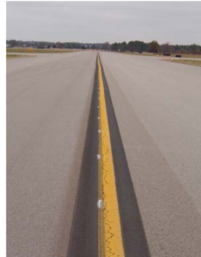
FIGURE 6-4. LAYOUT WITH PAINT SPOTS TO STRAIGHTEN EXISTING MARKINGS.
