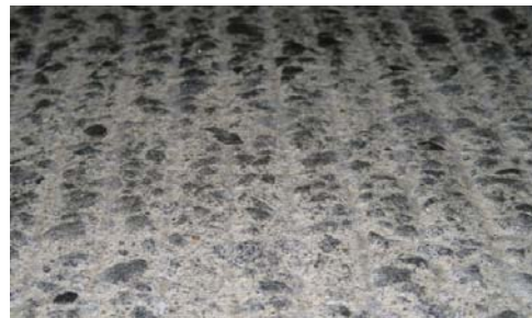
FIGURE 5-17. AFTER TEN YEARS OF SHOTBLASTING TO REMOVE RUBBER DEPOSITS.
