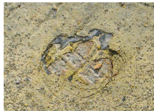
FIGURE 6-7. MULTIPLE LAYERS OF PAINT FILL THE GROOVES.
